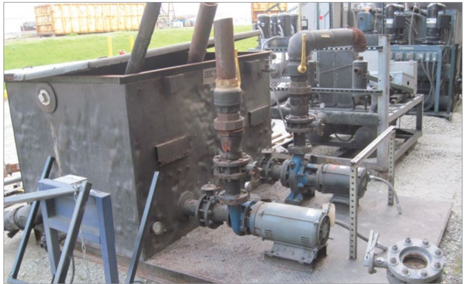
Old chilled water system equipment after removal.
