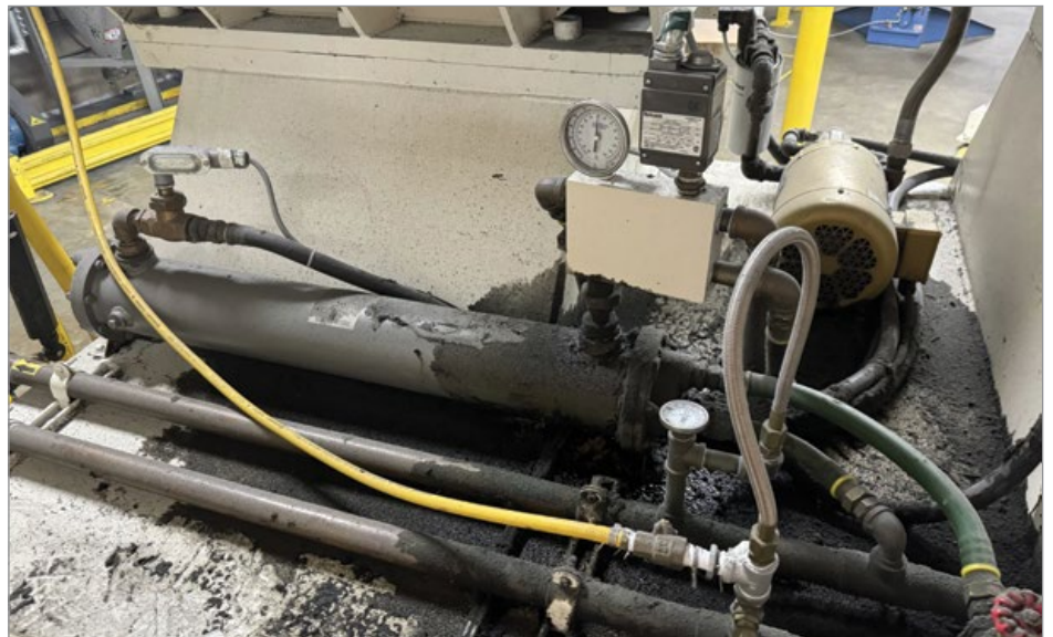
Gearbox oil cooler equipped with thermostatic control valve (in box with gauge) and leaving oil temperature sensor in fitting at other end of heat exchanger.
