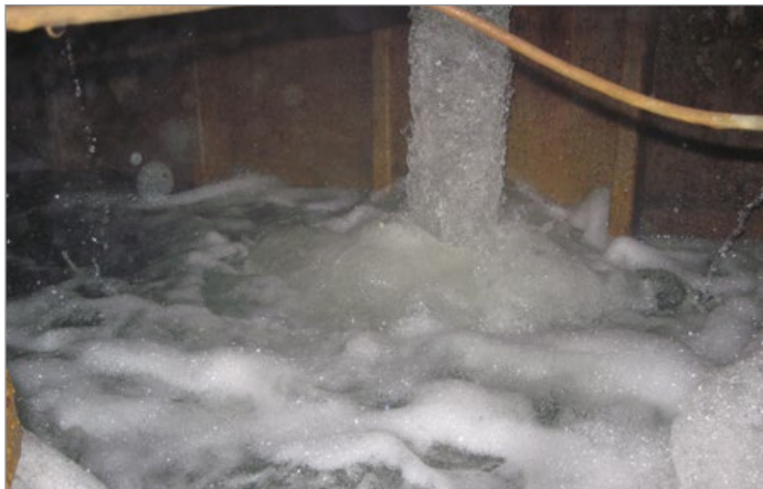
Highly aerated, free falling tower process return tank
