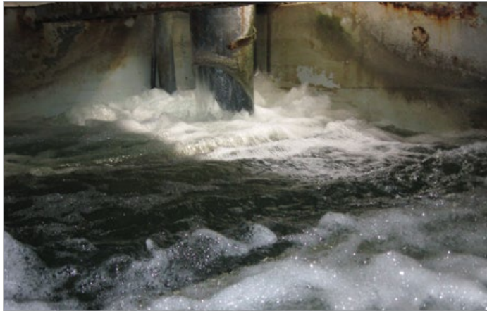
Typical highly aerated tower tank return
