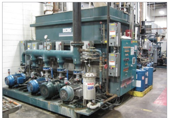
Typical Tower Water Tank System
