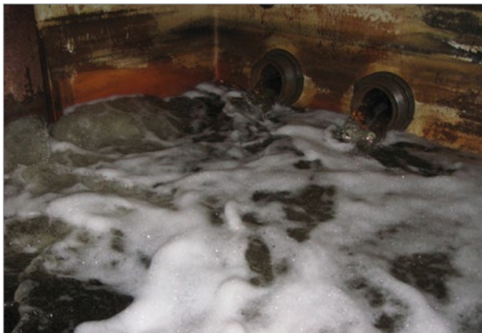
CHW hot well with aeration and balancing flow from cold well
