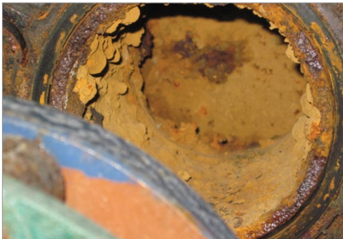
Chiller CHW inlet corrosion and deposits on tank system
