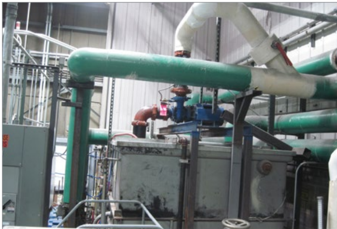
Pump added on top of chilled water tank
