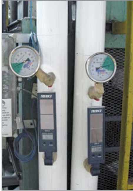
These gauges include decals showing the normal range of operation.
