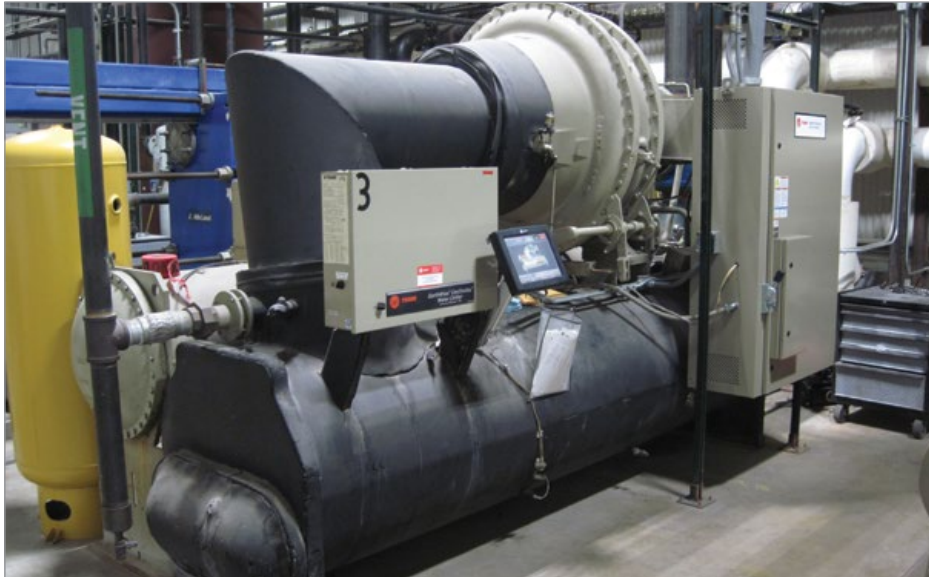
A 400 ton centrifugal chiller with VFD retrofit.
