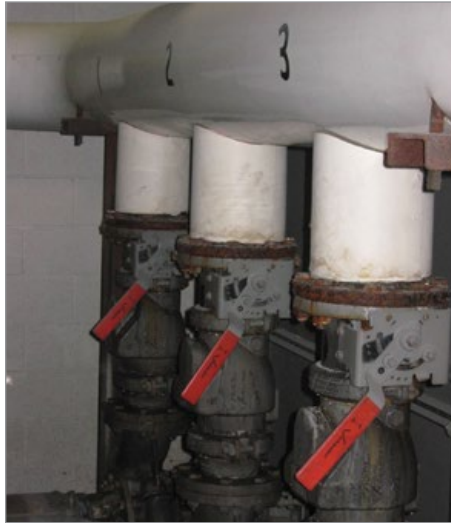
Partially closed chilled water pump discharge valves.
