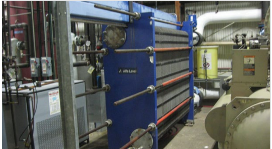
Free cooling plate heat exchanger.
